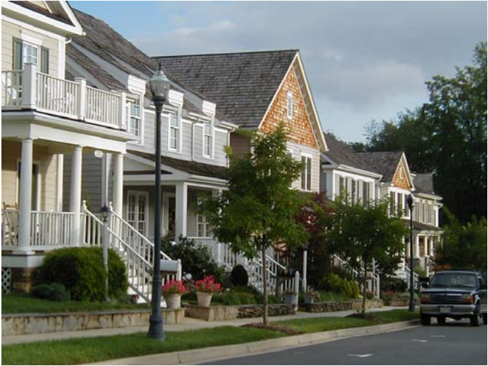
Development within the first block on either side of Tamiami Trail should be residential in character and relatively dense.
